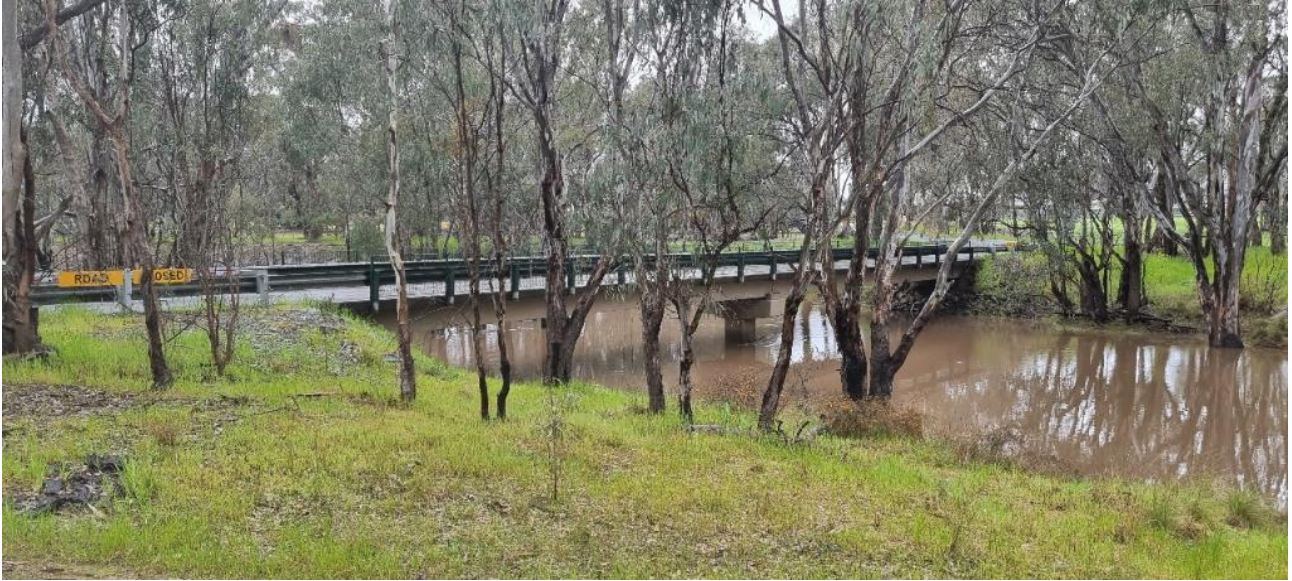
Figure 88 – Raftery Road bridge over Sevens Creek, Shepparton
