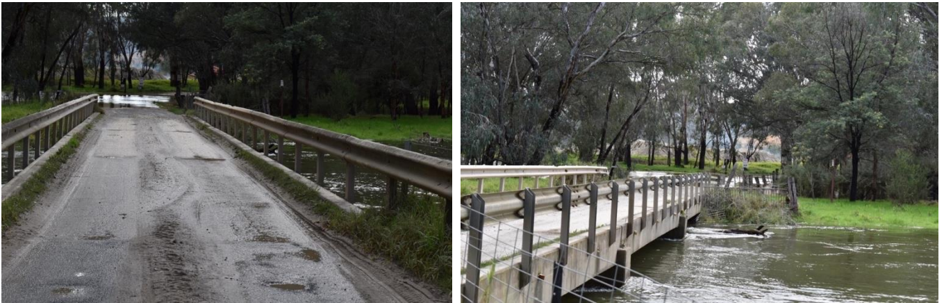
Figure 89 – Inundation of approach to Carrolls Lane Bridge, Wodonga
