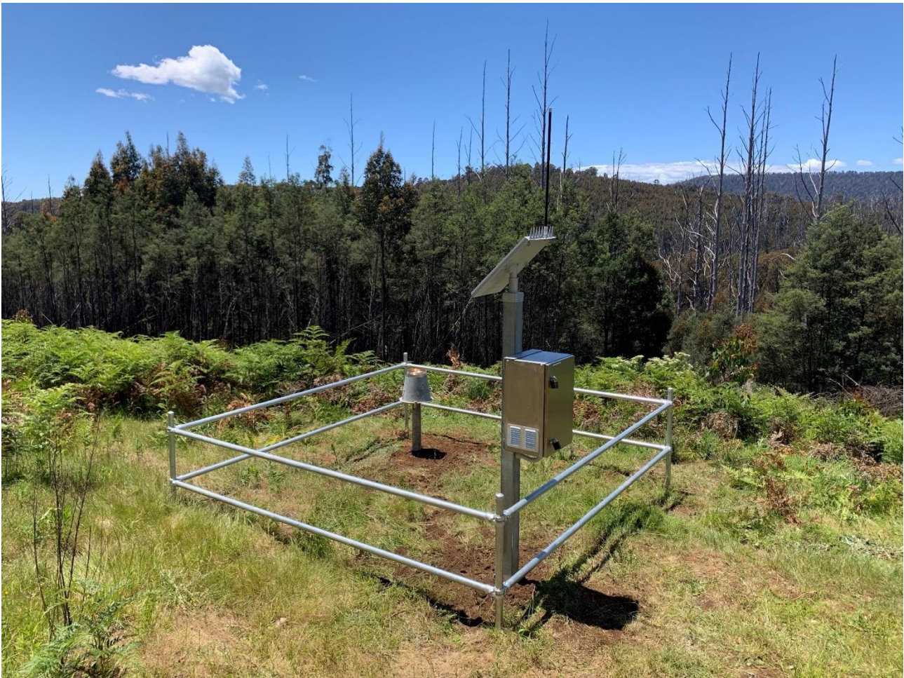
Figure 98 – Upper Murrindindi Rainfall gauge installed as part of the Victorian CMP, Ventia, December 2022
