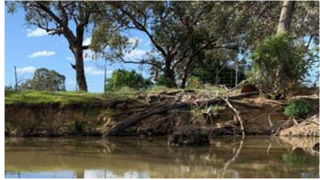
Figure 98: Bank Erosion on Gunbower Creek (photo courtesy of A Hodge)
