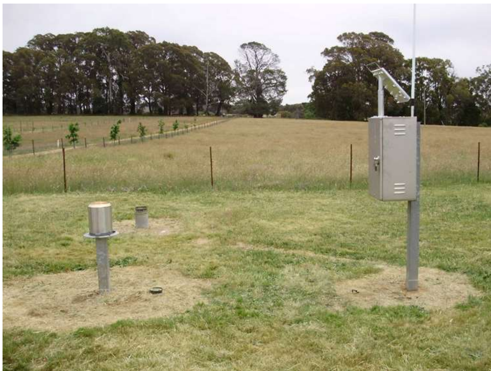
Figure 16 Rain gauge installation at Strathbogie Ranges
