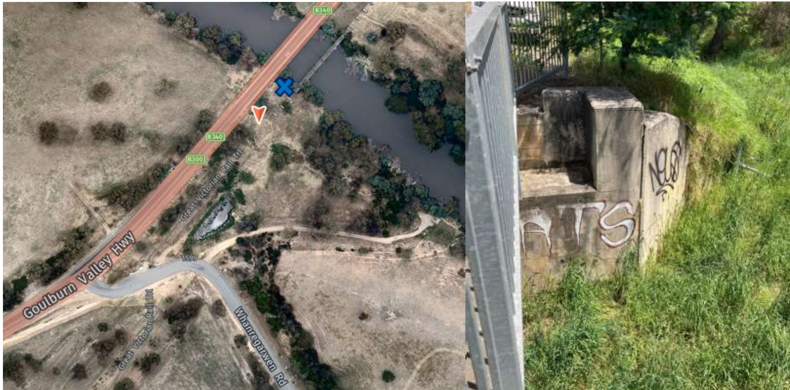
Figure 17 Location Map & Site Photo - 1. Goulburn River at Molesworth: Streamflow Gauge
