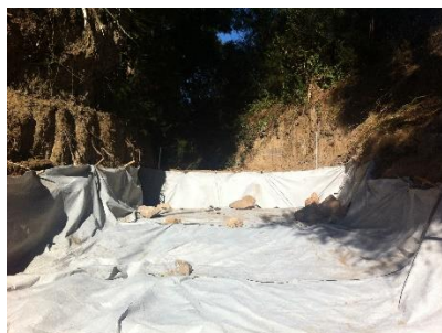
Figure 80. Application of geotextiles (Source: S. Clevon).
