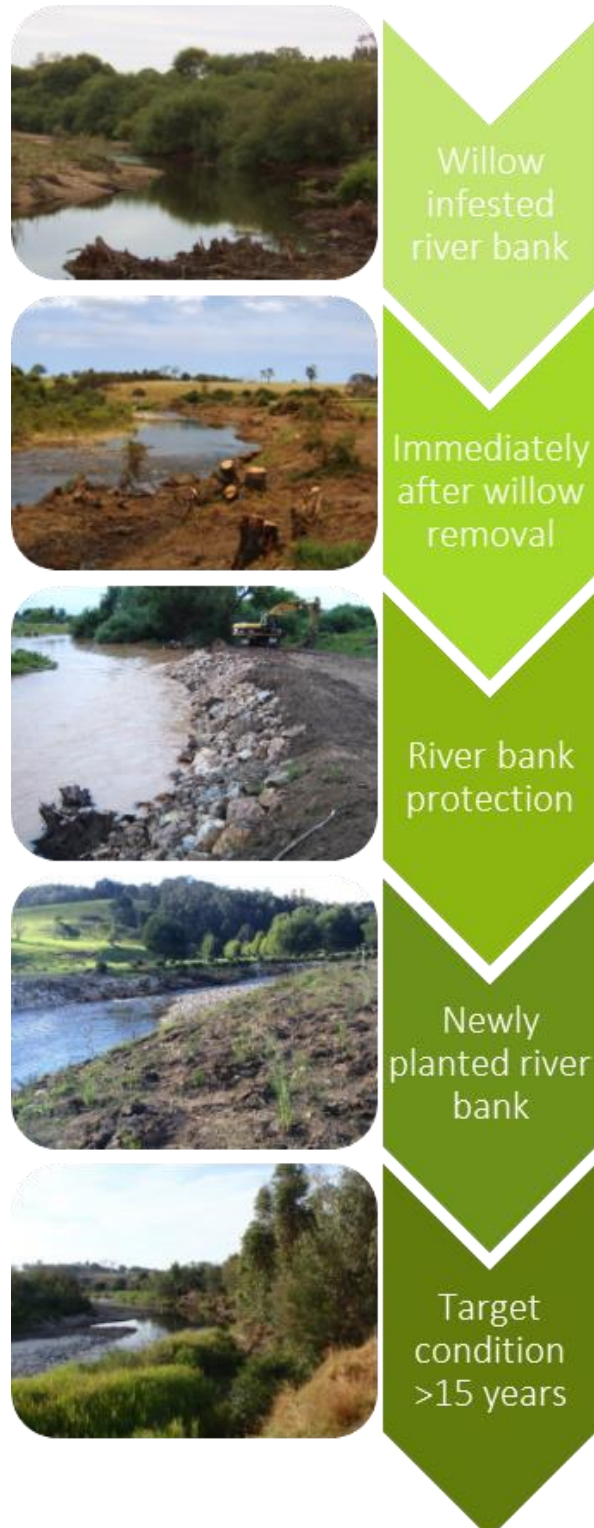
Figure 50. Approach for approach for willow replacement, management of willow debris and bank stabilisation.
