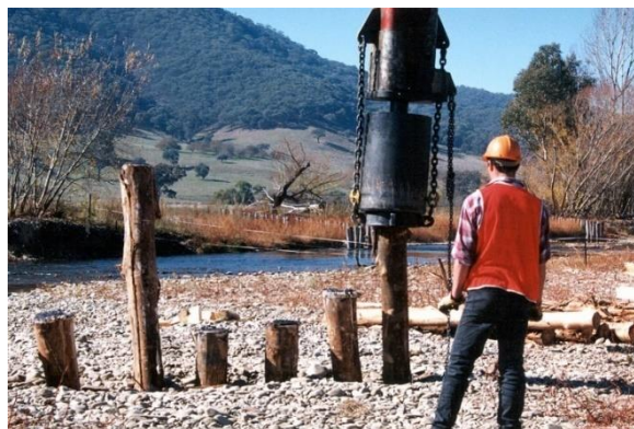
Figure 77. Timber piles in north east Victoria (Photo courtesy of North East CMA).
