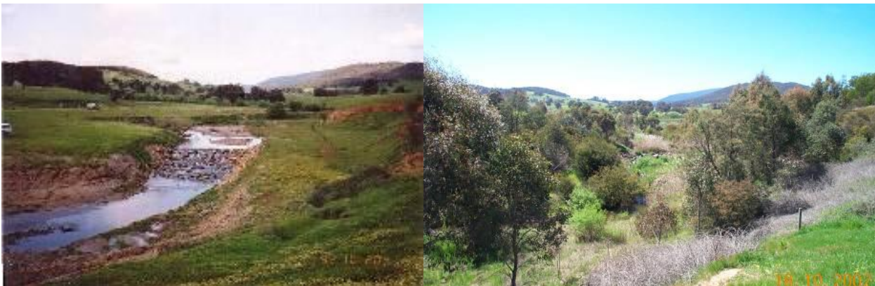
Figure 70. Barwidgee Creek, north east Victoria, six months (left) and 10 years (right) after rock chute construction and revegetation (Images courtesy of T. McCormack, North East CMA).
