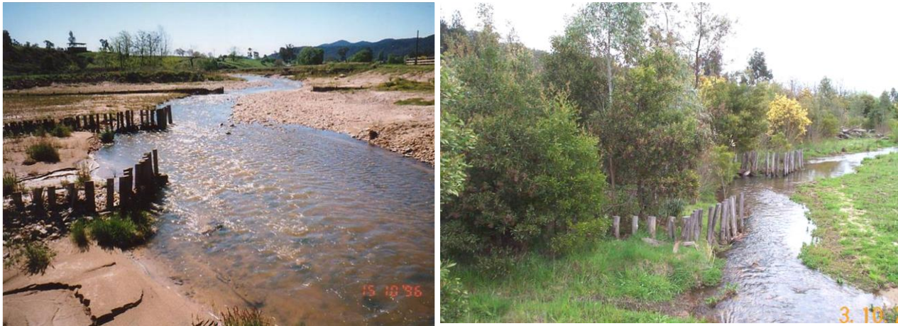
Figure 55. Example of vegetation establishment within the embayment's of pile fields at Black Range Creek in north east Victoria.
