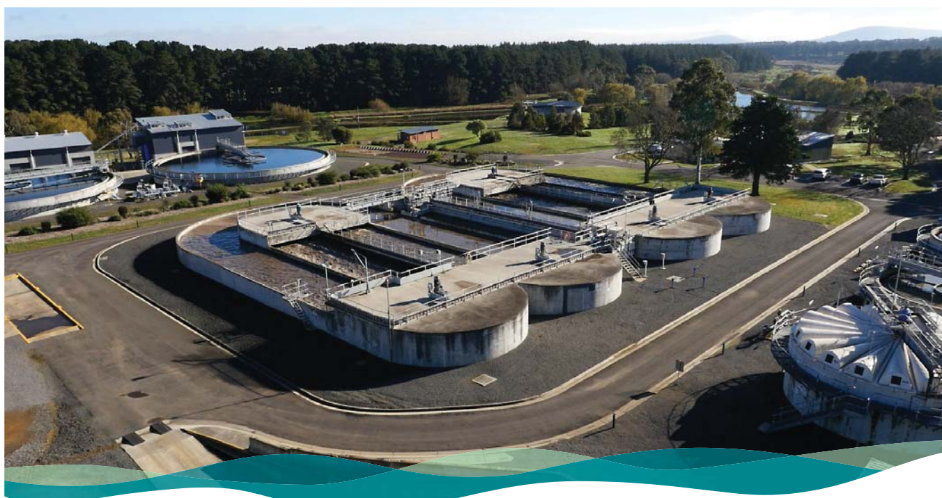
Ballarat North Wastewater Treatment Plant. Courtesy: Central Highlands Water
