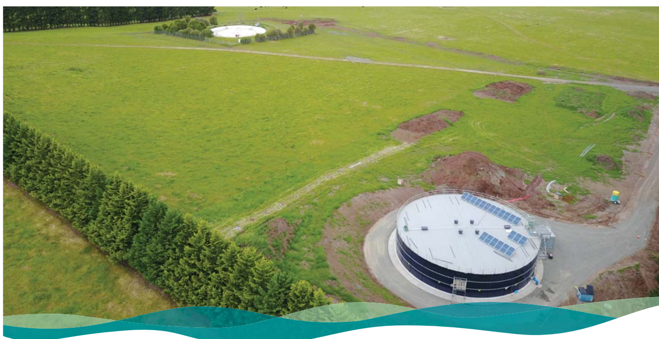
Ballan new tank and old basin. Courtesy: Central Highlands Water
