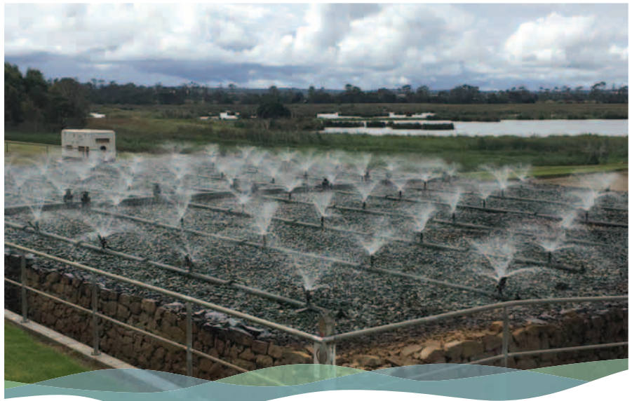
Bairnsdale waste water treatment plant. Courtesy: East Gippsland Water
