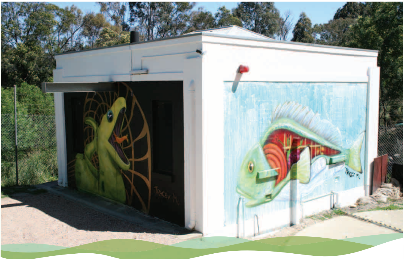
Transforming a pump station with Aboriginal-inspired art. Courtesy: East Gippsland Water
