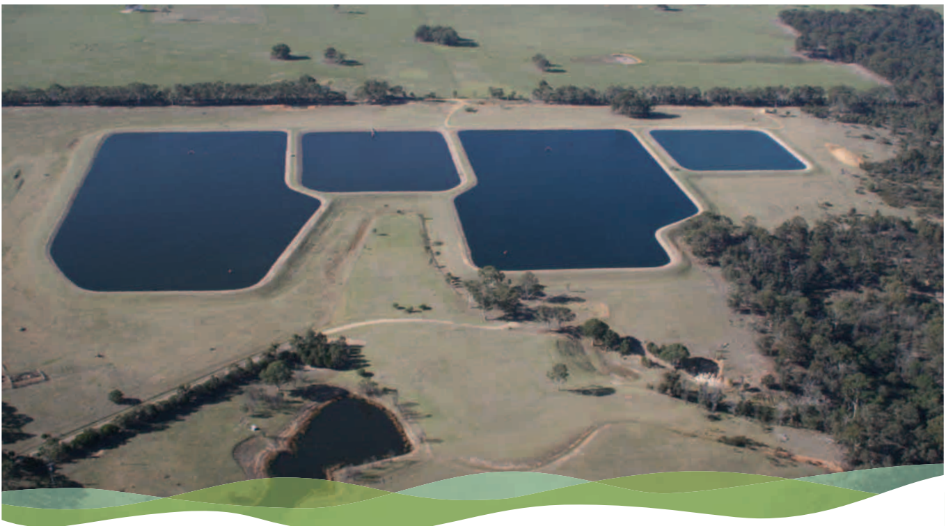
Paynesville wastewater storage lagoons. Courtesy: East Gippsland Water
