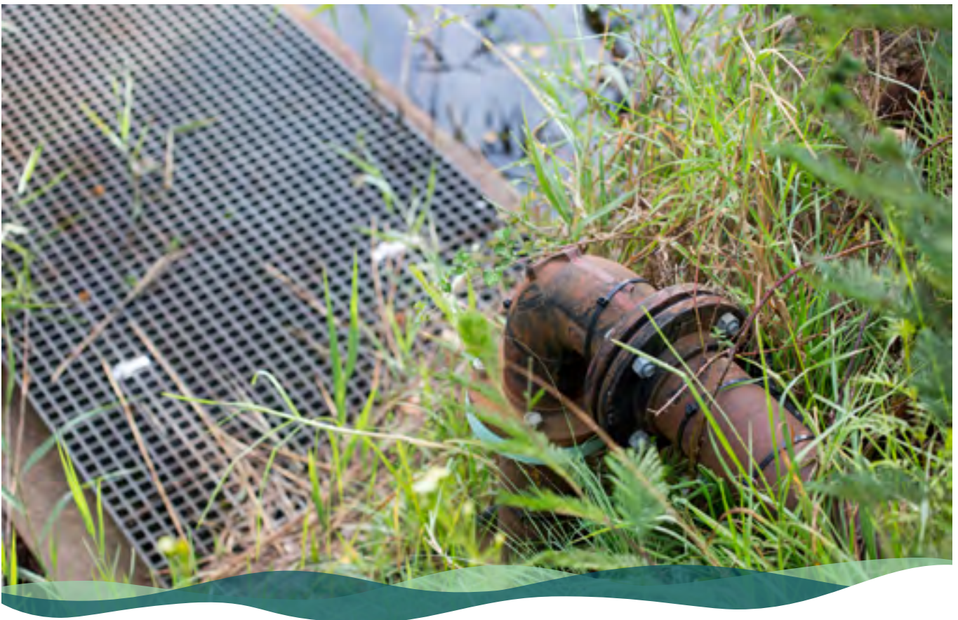
Bemboka Treatment Plant. Courtesy: Wimmera CMA
